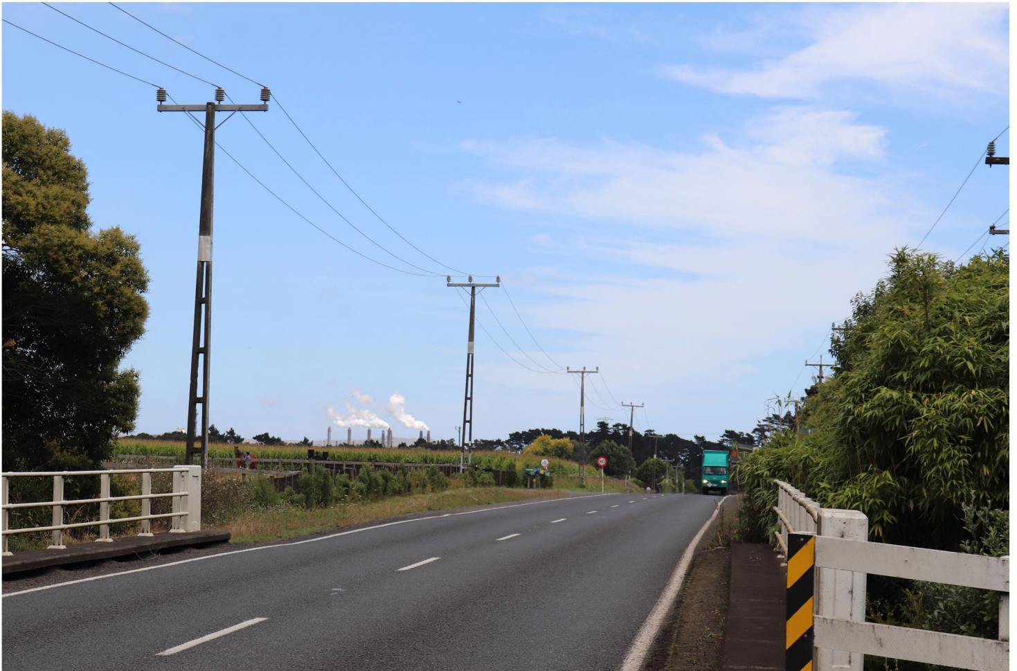
Photo Viewpoint 15 - 40 Brookside Road, Glenbrook
